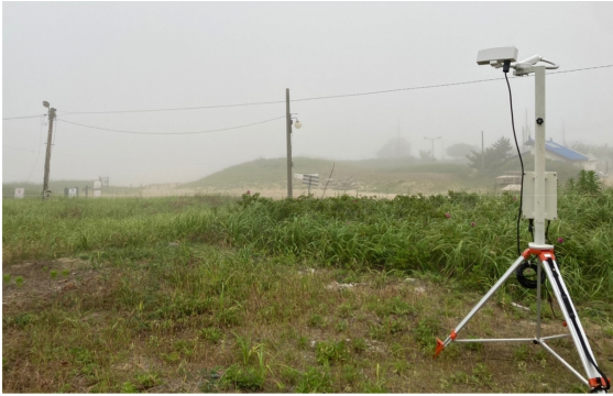
Fig. 4. The installed visibility measurement instrument (PWD20) in the observation site (Hagampo).
